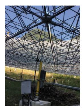
Fig. 2: One actuator connected to its node plate.
